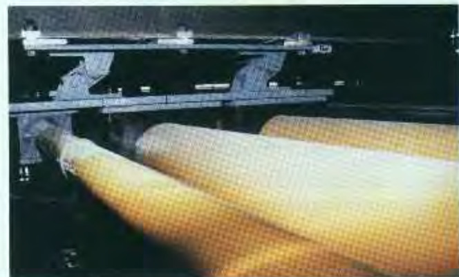
Fig. 194: Pipe support with flexible mountings for isolating structure-borne sound
