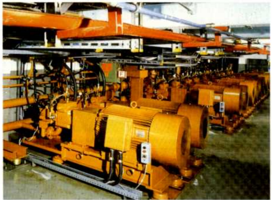
Fig. 148: Central oil supply, motor-pump stations
